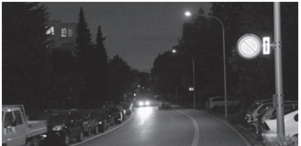
LED-Strassenlampen an Gandstrasse.
